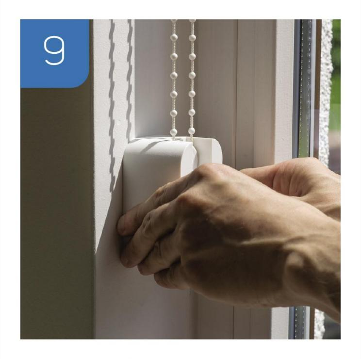
Attach the Smart Shades to the wall. Use the tape on the back of the device or screws (not included). Make sure that the chain is not crossed or too loose. See the following images.
